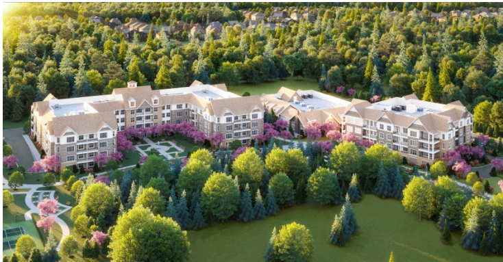
Rendering of Fountaingate Gardens Life Plan Community located on the Gurwin Healthcare System campus in Commack, NY.
